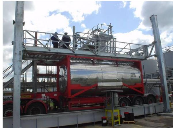
Both ISO-containers and round barrel tankers can be accessed. The floor prevents operators walking off the end of the tanker
