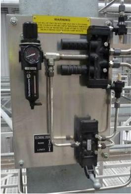
TCEN4's are pneumatically powered and require 5.5 barg for efficient operation.
