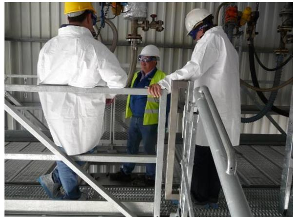
The cage provides a safe and clean working environment where loading arms and hoses can be easily deployed
