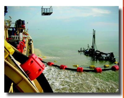
The colour pigment is moulded-in and consequently not added as a coating ensuring greater life of the colour and a big help to the environment as it never requires additional paintings, avoiding toxic dispersions in the water. Floatex polyethylene require a minimal maintenance.
